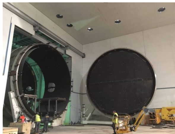
On site Installation
