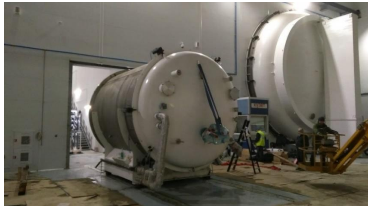
On site installation
